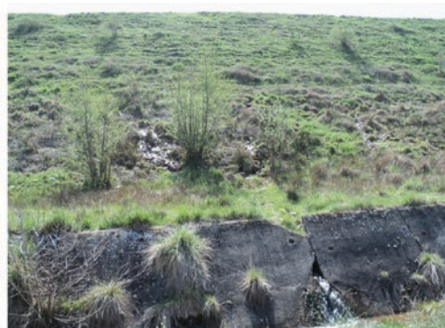
Seepage springs and slope instability
