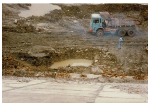
Seepage chimney at the upstream toe
